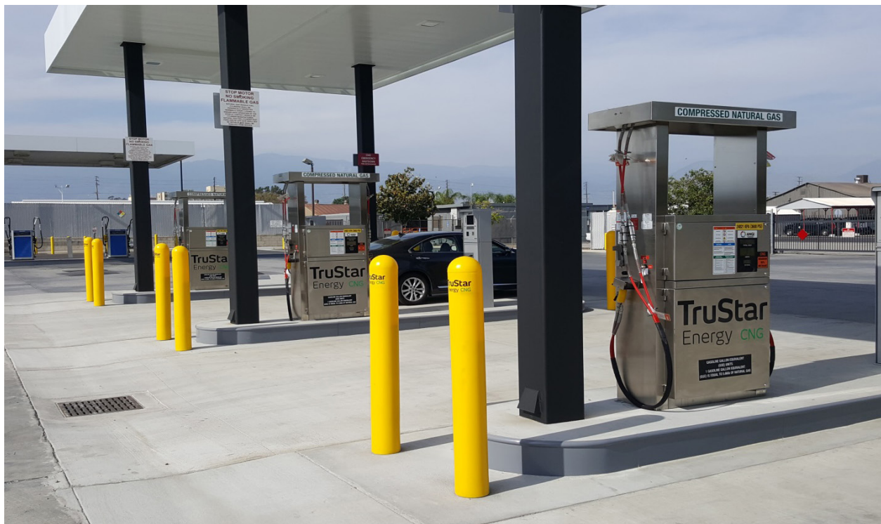
TruStar Fuel Station at City Yard
